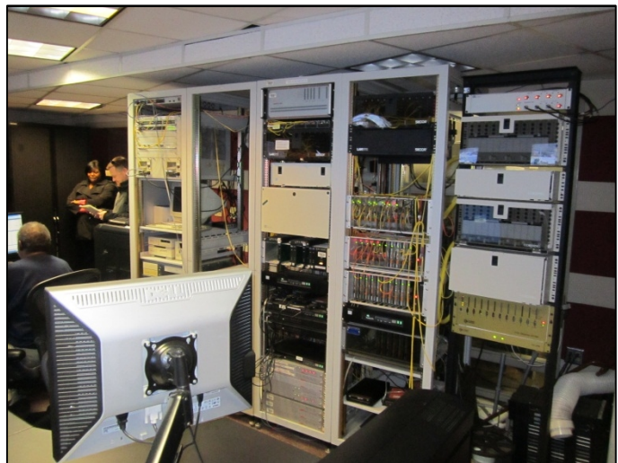
Figure 5-7: TCC Signal Controllers
